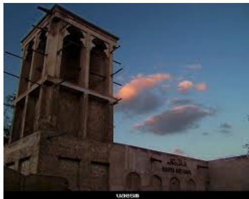
Badgers used for catching air and cooling with natural ventilation in Islamic architecture
